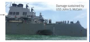
Damage sustained by USS John S. McCain
